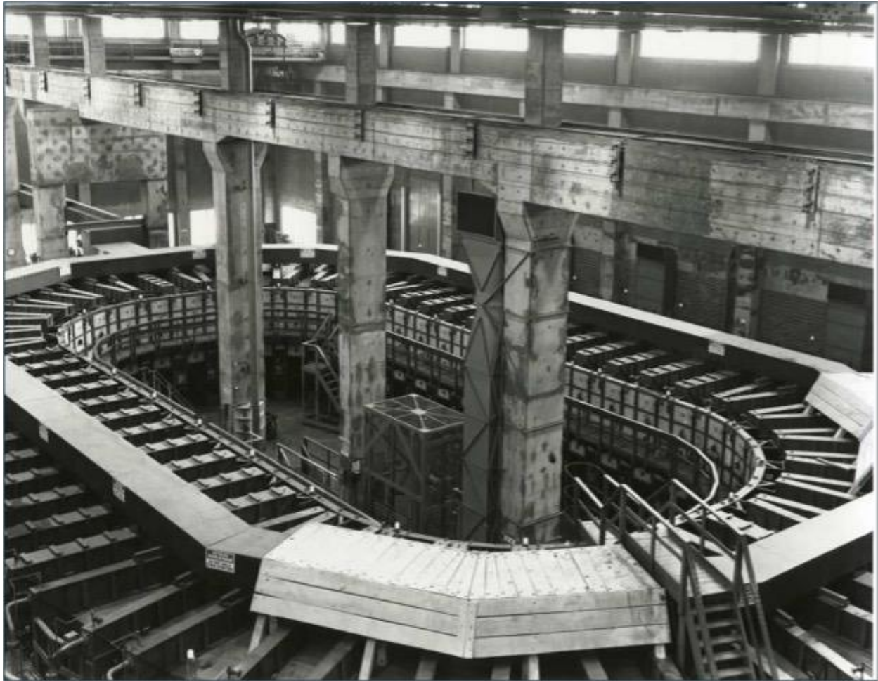
The Y-12 Electromagnetic Processing Plant's 'racetrack'. Clinton Engineer Works, Oak Ridge TN. Photo by Ed Westcott (Public domain Courtesy of Barbara Scollin)
